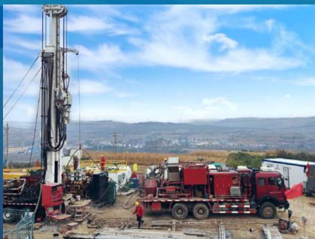
ZX-SH-UM15V/H井组远端对接井施工现场
